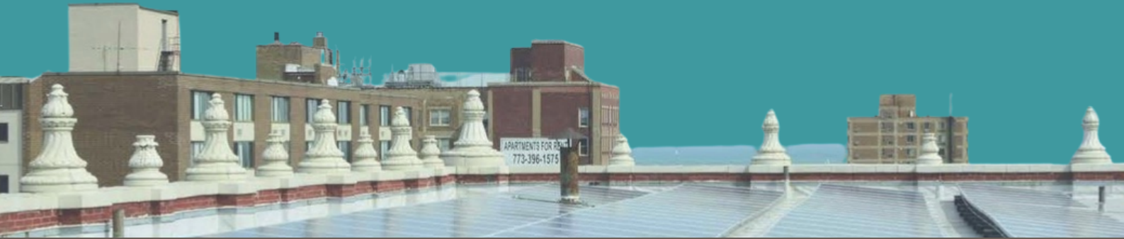
ICA GreenRise has 483 solar panels, providing 25% of the building's electricity; some panels pictured here.
